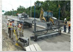
The project consisted of two three-lane bridge approaches. The 193 individual slabs were installed between slipformed sections of new highway and two existing bridges. Normal weight precast concrete Super-Slab® panels were used for full-depth replacement on the roadway. Work was completed during four separate weekends while traffic was detoured to the other side of the divided highway. High-production dual-slope Supergrading was done using a laser-guided Somero S-240.
